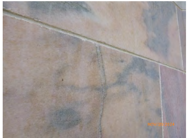
130-74 Stone_Crack Repair sound 2024-3.jpg
