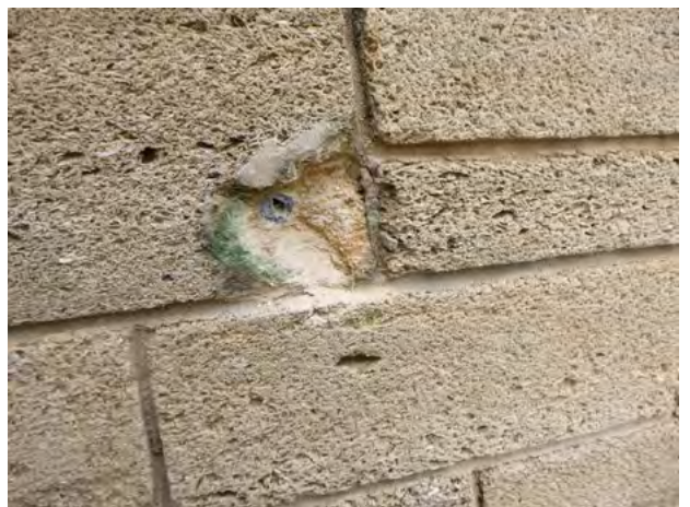
162-15 Stone_Repair Patch Removed 2024-1.jpg
