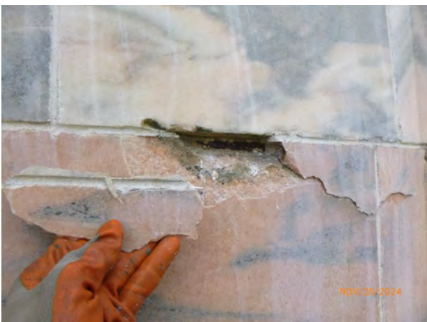
132-71 Stone_Spall Removed + Steel 2024-2.jpg
