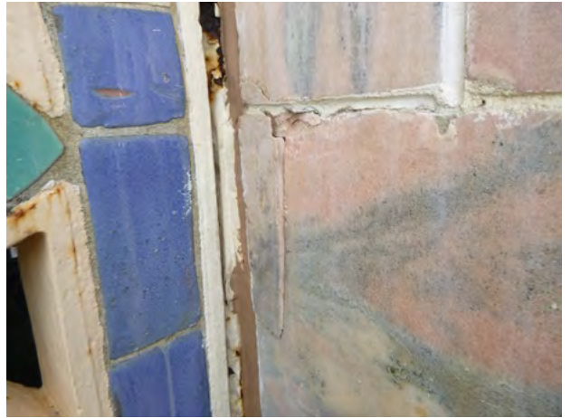
41-172 Stone_Spall Bonded 2024-1.jpg
