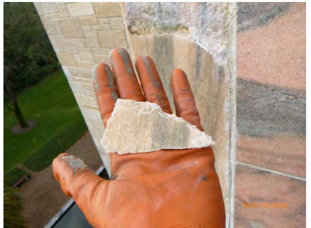
241-57 Stone_Spall Removed + Steel 2024-4.jpg
