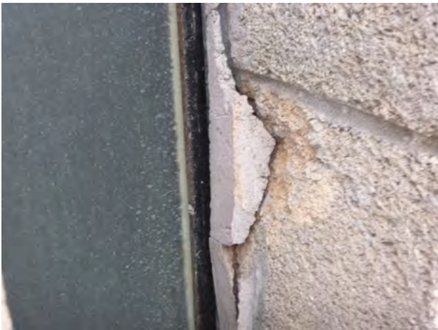
51-87 Stone_Spall Removed + Steel 2024-1.jpg
