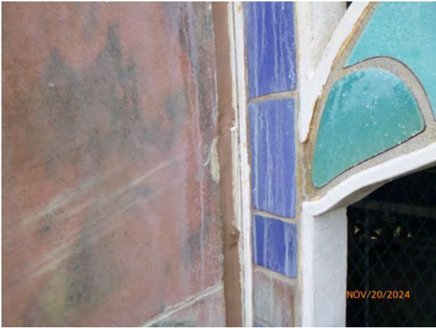
136-153 Stone_Repair Patch Sound 2024-1.jpg
