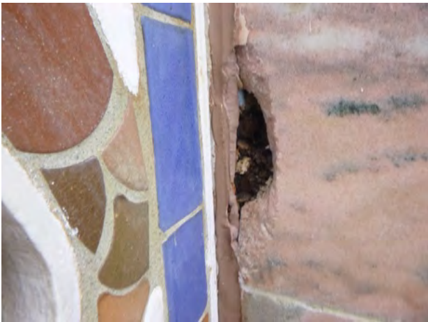
194-154 Stone_Spall Removed + Steel 2024-4.jpg
