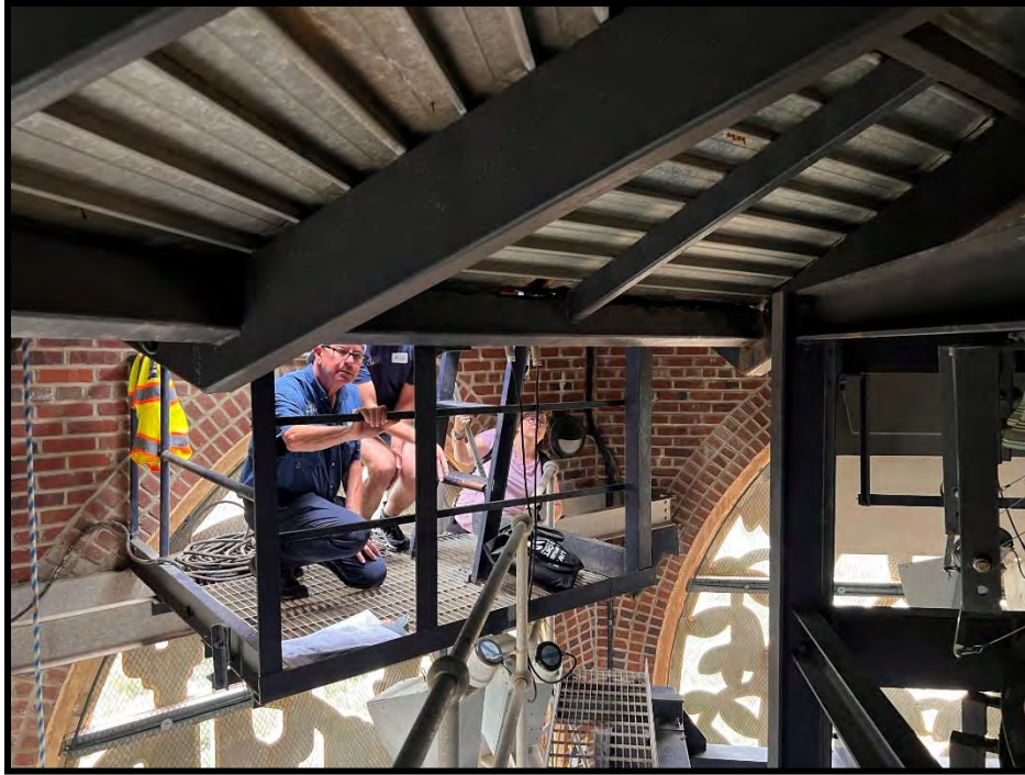
Figure 6 Upper roof framing
