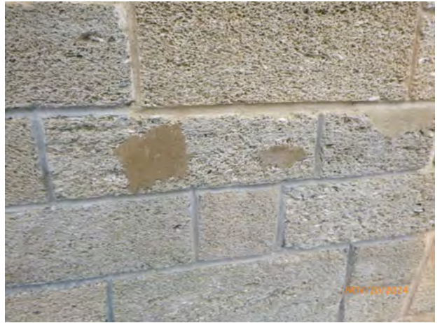
64-70 Stone_Repair Patch Sound 2024-1.jpg
