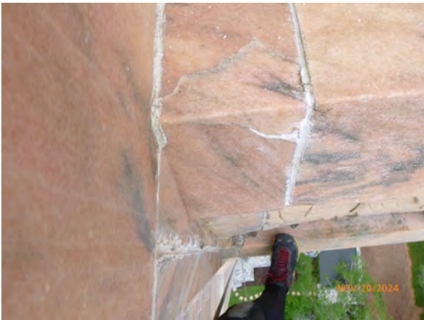
133-141 Stone_Spall Bonded 2024-3.jpg
