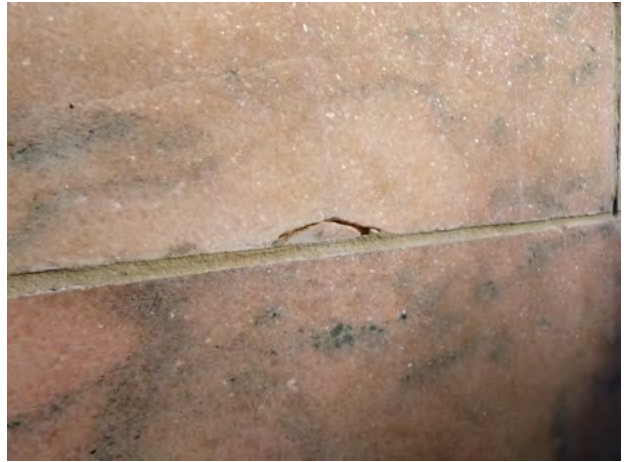
257-28 Stone_Spall Bonded 2024-1.jpg
