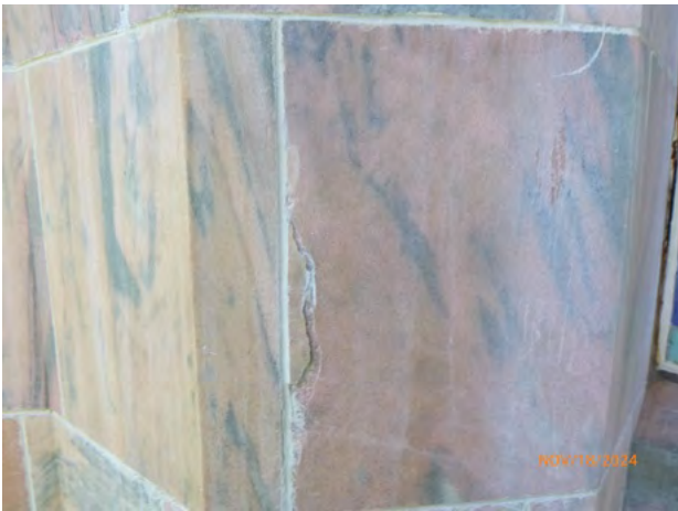
33-146 Stone_Spall Bonded 2024-1.jpg
