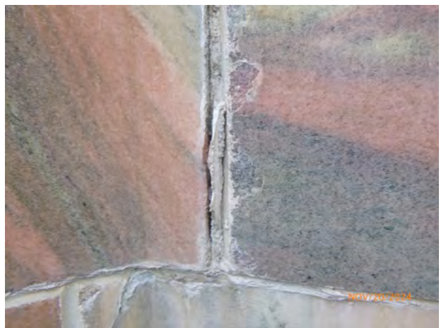
132-181 Stone_Joints Mortar Removed 2024-2.jpg
