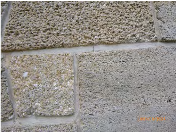
366-55 Stone_Crack System units and joints 2024-5.jpg
