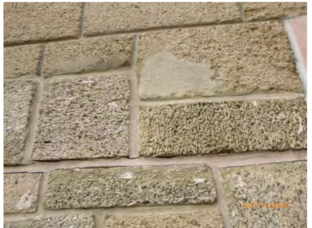
239-91 Stone_Repair Patch Sound 2024-1.jpg
