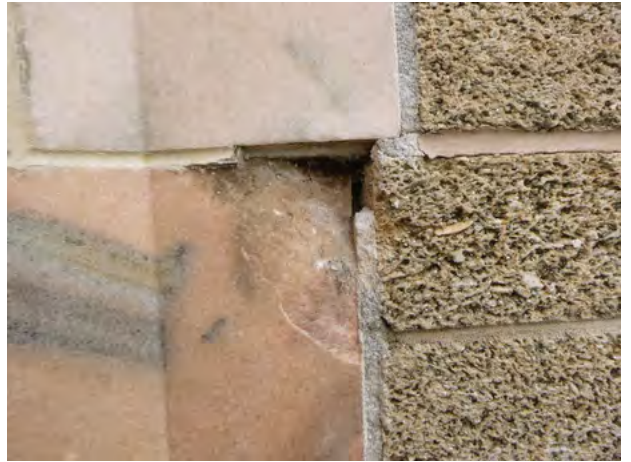
160-66 Stone_Spall Removed + Steel 2024-2.jpg
