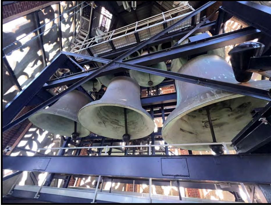
Figure 7 Carillon steel support frame
