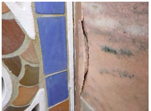
194-154 Stone_Spall Removed + Steel 2024-1.jpg
