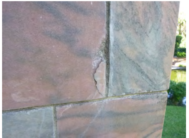
373-15 Stone_Spall Bonded 2024-1.jpg
