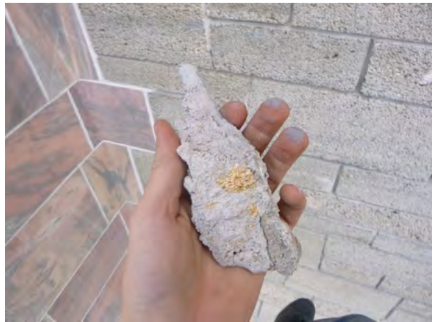
51-87 Stone_Spall Removed + Steel 2024-2.jpg
