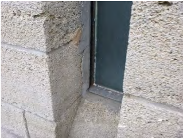
50-87 Stone_Spall Bonded 2024-2.jpg
