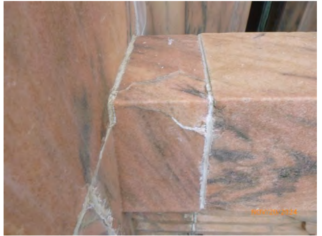
133-141 Stone_Spall Bonded 2024-2.jpg
