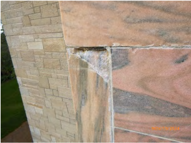
241-57 Stone_Spall Removed + Steel 2024-1.jpg
