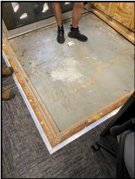
Figure 23 Hatch in the Library floor build up, water passes through storefront to reach interior drains
