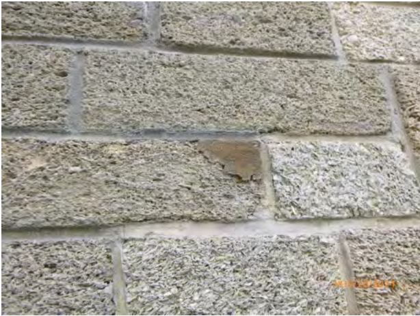
63-83 Stone_Repair Patch Sound 2024-1.jpg
