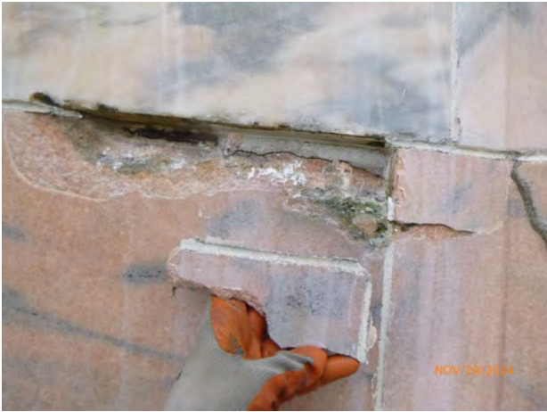
132-71 Stone_Spall Removed + Steel 2024-4.jpg
