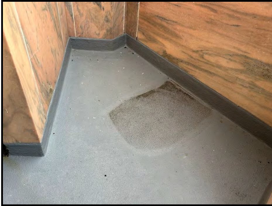
Figure 42 Cracked roof membrane at the low roof
