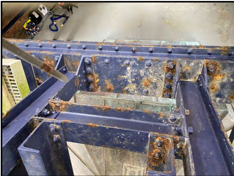
Figure 31 Carillon framing above the Playing Cabin, viewed from above.
