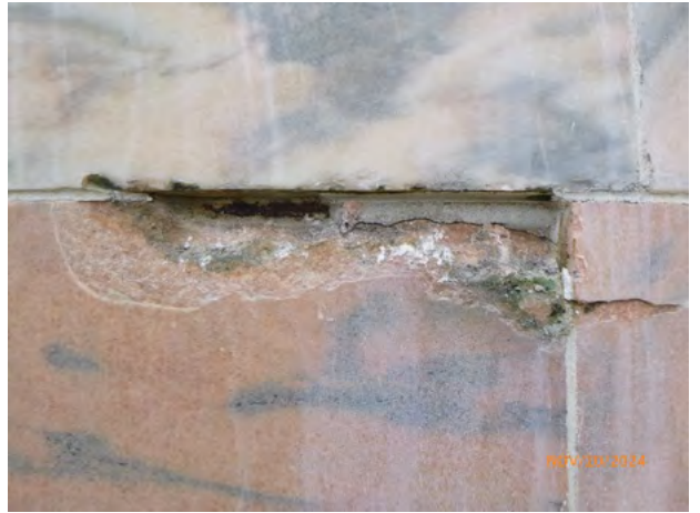
132-71 Stone_Spall Removed + Steel 2024-5.jpg
