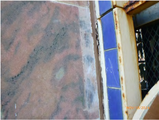
380-154 Stone_Repair Dutchman Sound 2024-3.jpg
