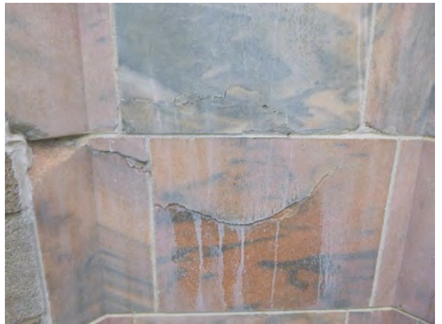
141-69 Stone_Spall Removed + Steel 2024-1.jpg
