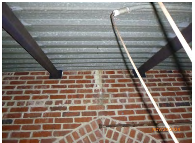
651-182 Brick_SoilStain Paint 2024-1.jpg
