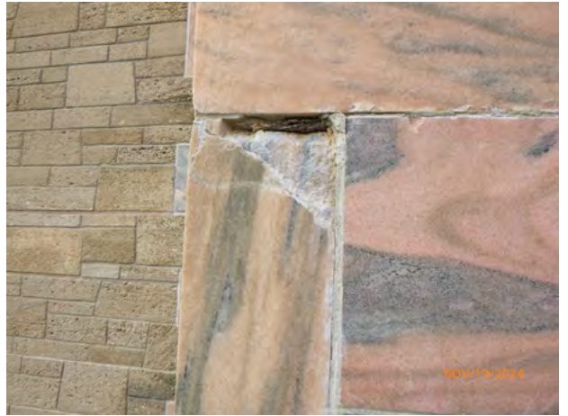
241-57 Stone_Spall Removed + Steel 2024-2.jpg
