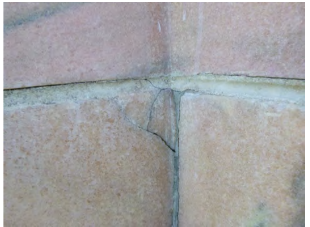
35-138 Stone_Spall Bonded 2024-1.jpg
