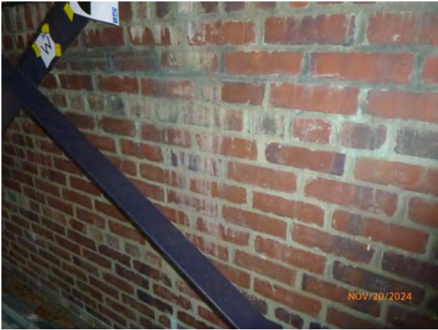
652-139 Brick_SoilStain Paint 2024-1.jpg
