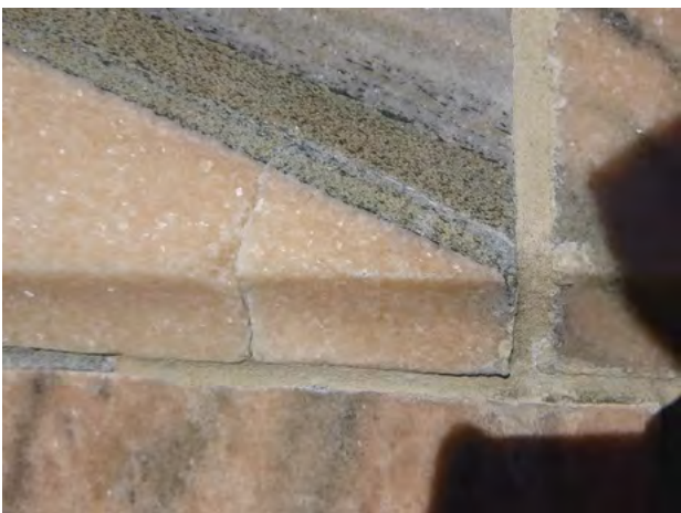
335-184 Stone_Spall Bonded 2024-1.jpg
