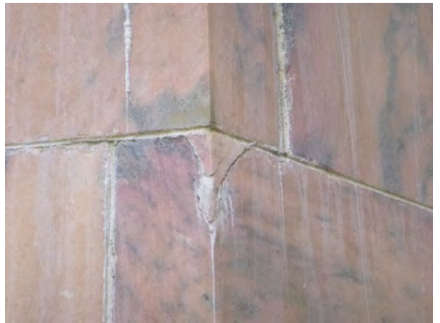
79-161 Stone_Spall Bonded 2024-1.jpg
