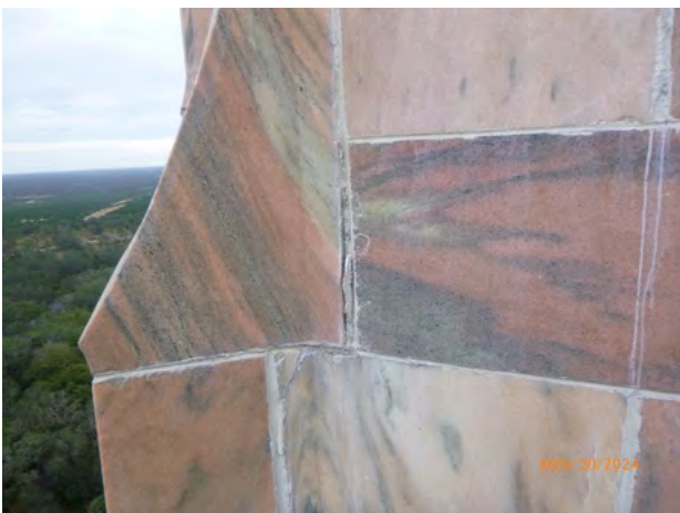
132-181 Stone_Joints Mortar Removed 2024-1.jpg
