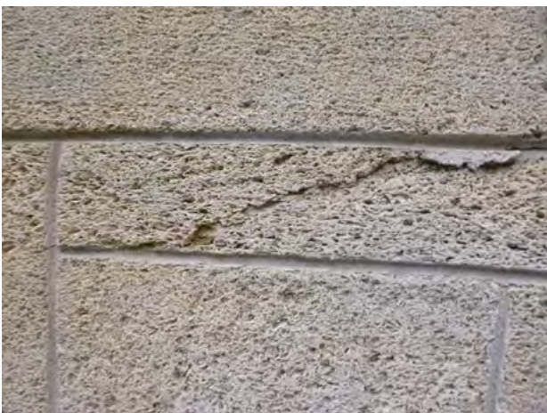
137-15 Stone_Spall Bonded 2024-1.jpg
