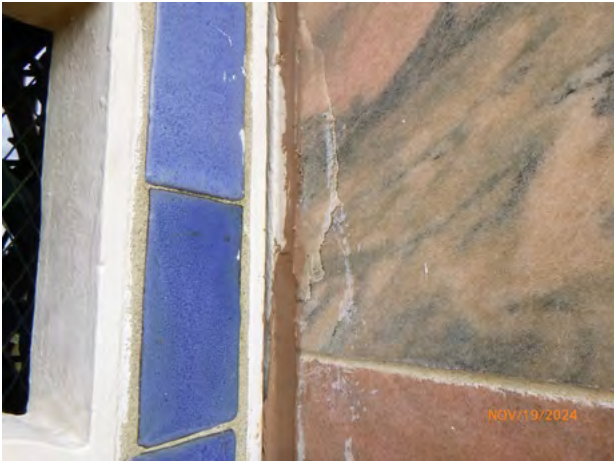
222-153 Stone_Spall Bonded 2024-2.jpg
