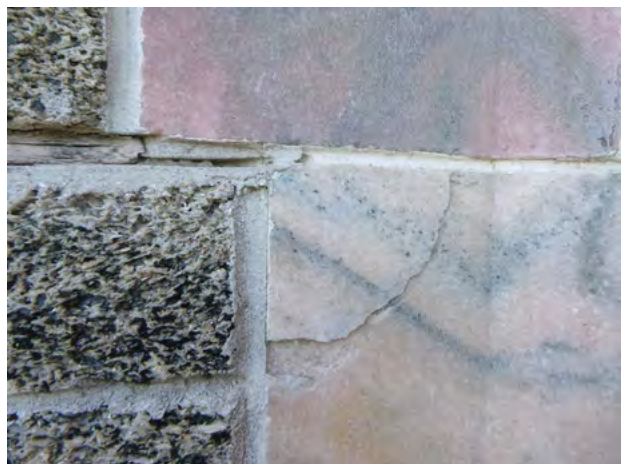
40-82 Stone_Spall Bonded 2024-1.jpg
