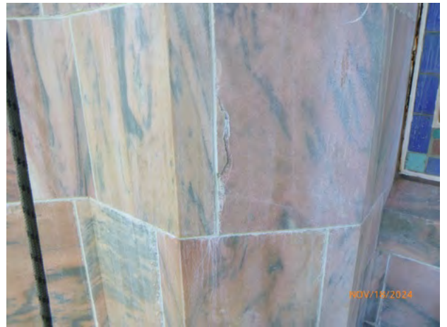
33-146 Stone_Spall Bonded 2024-2.jpg
