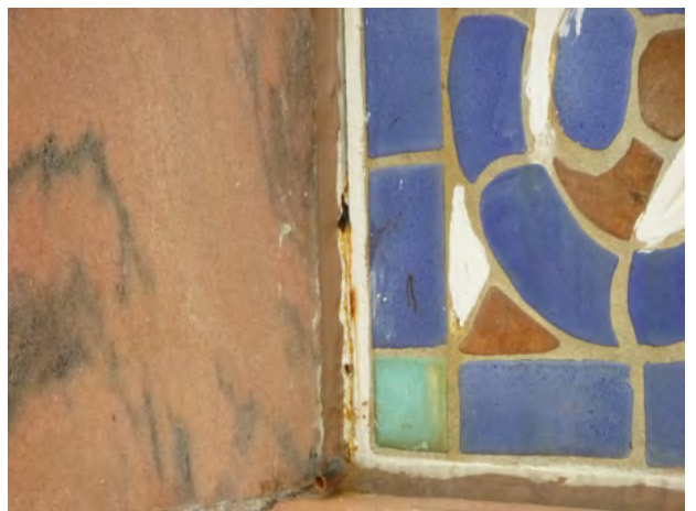
182-146 ArchMetal_Corrosion Pitted 2024-1.jpg
