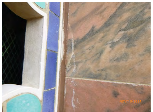
222-153 Stone_Spall Bonded 2024-1.jpg
