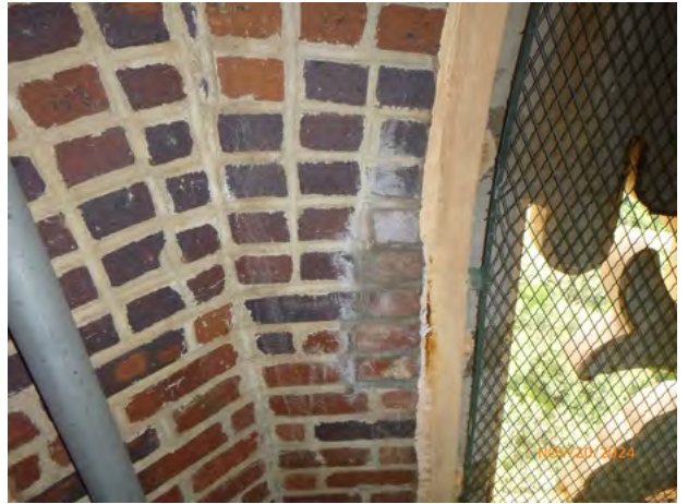
847-172 Brick_Repair Patch Sound 2024-1.jpg
