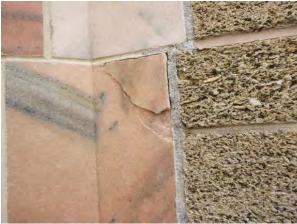
160-66 Stone_Spall Removed + Steel 2024-1.jpg
