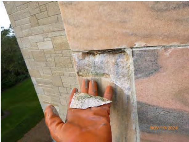
241-57 Stone_Spall Removed + Steel 2024-3.jpg
