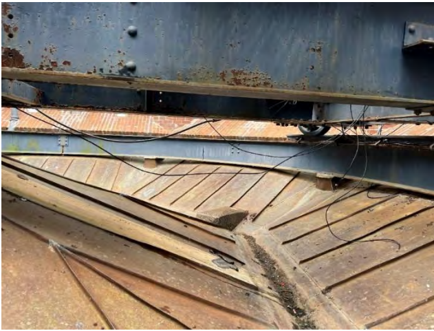
2 Upper Roof. Single drain visible.
