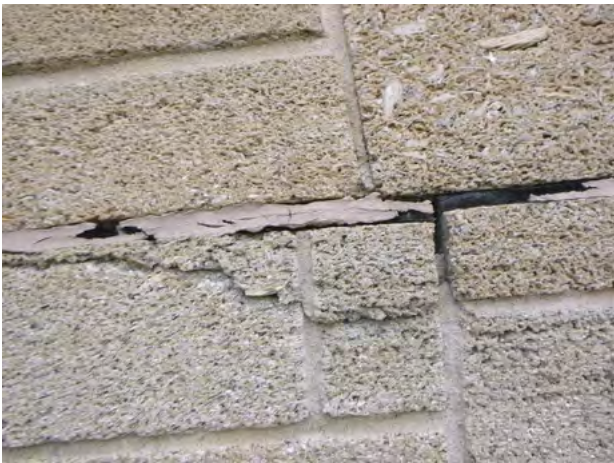
149-91 Stone_Spall Removed + Steel 2024-1.jpg
