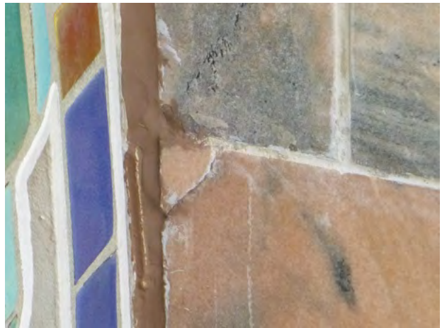
194-171 Stone_Spall Bonded 2024-1.jpg
