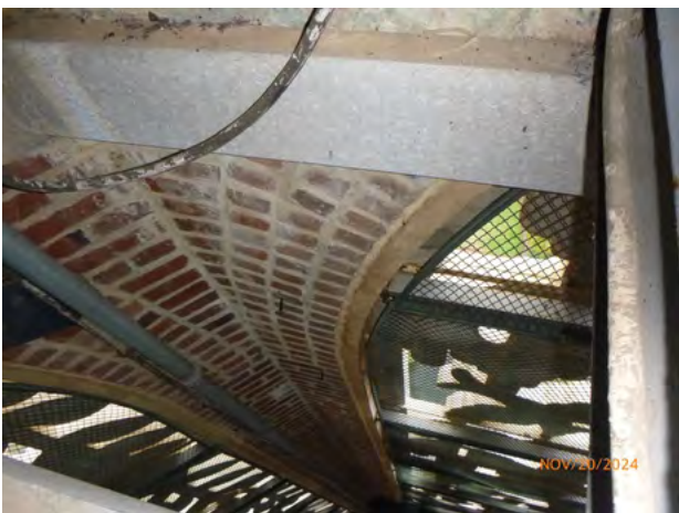
542-171 Brick_SoilStain Paint 2024-1.jpg
