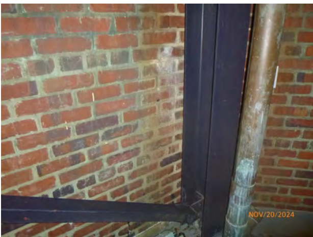
656-140 Brick_SoilStain Paint 2024-1.jpg
