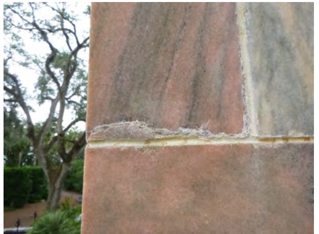
228-18 Stone_Spall Bonded 2024-1.jpg
