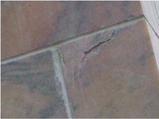
55-85 Stone_Spall Bonded 2024-1.jpg
