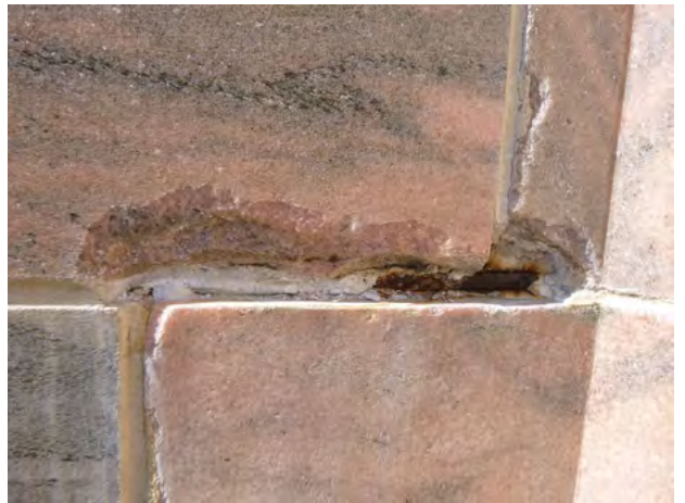
328-50 Stone_Spall Removed + Steel 2024-2.jpg
