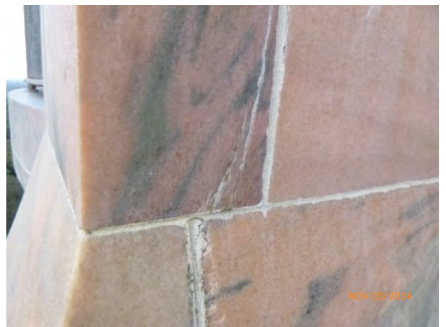
130-123 Stone_Crack Repair sound 2024-2.jpg
