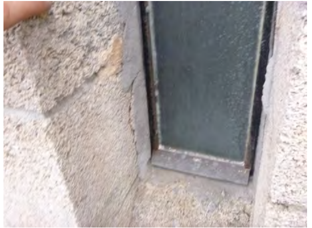
50-87 Stone_Spall Bonded 2024-1.jpg
