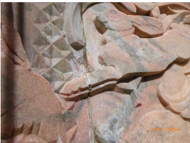
273-30 Stone_Spall Missing 2024-1.jpg
