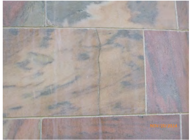
130-74 Stone_Crack Repair sound 2024-1.jpg
