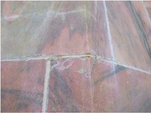
42-171 Stone_Spall Bonded 2024-1.jpg
