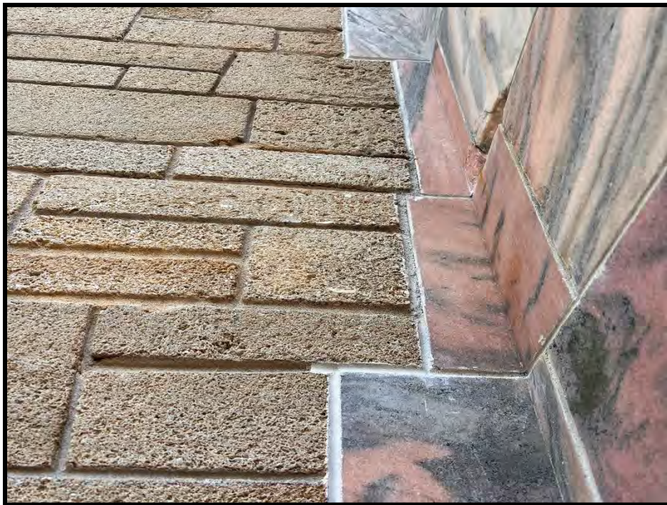
Figure 3 Exterior coquina stone (left) and pink Georgia Etowah marble (right)
