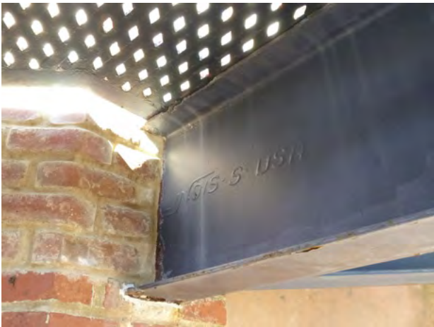
532-193 ArchMetal_Corrosion Surface 2024-1.jpg
