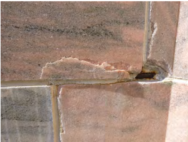
328-50 Stone_Spall Removed + Steel 2024-1.jpg
