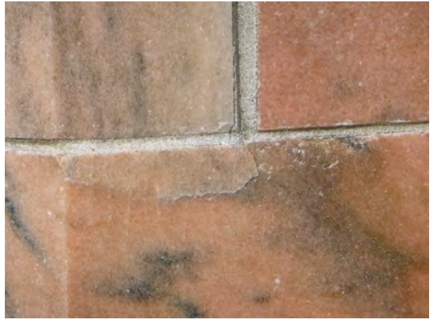
234-187 Stone_Spall Bonded 2024-1.jpg
