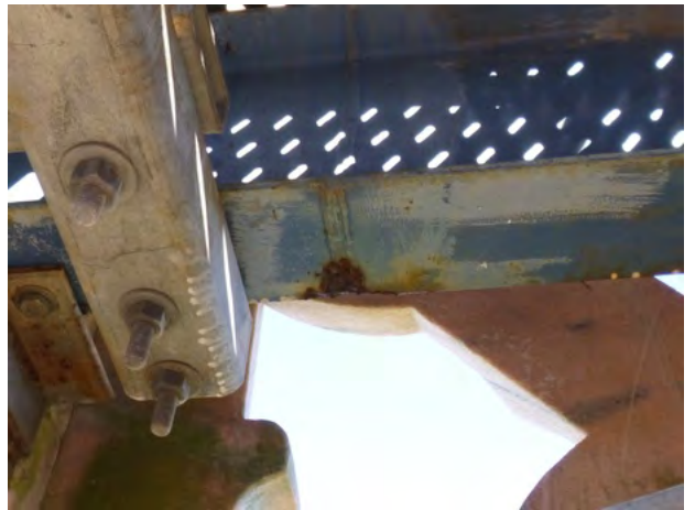
549-193 ArchMetal_Corrosion Surface 2024-1.jpg
