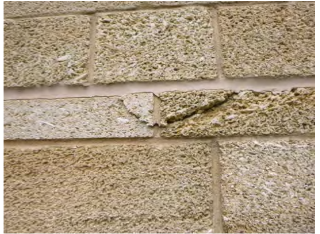
163-38 Stone_Spall Bonded 2024-1.jpg
