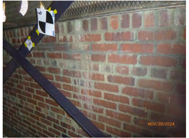
652-139 Brick_SoilStain Paint 2024-2.jpg
