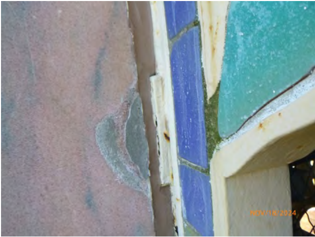
36-154 Stone_Spall Bonded 2024-3.jpg
