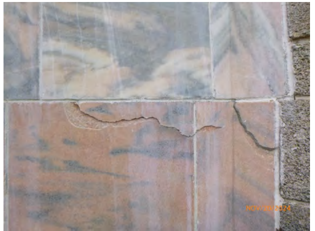
132-71 Stone_Spall Removed + Steel 2024-1.jpg
