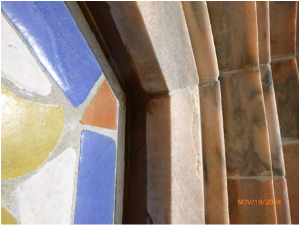
239-178 Stone_Spall Bonded 2024-3.jpg
