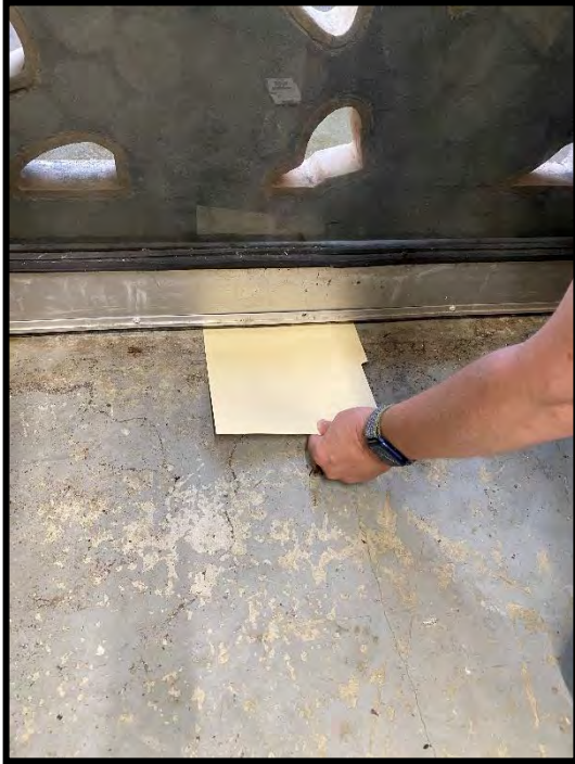
Figure 24 Demonstration of unsealed storefront
