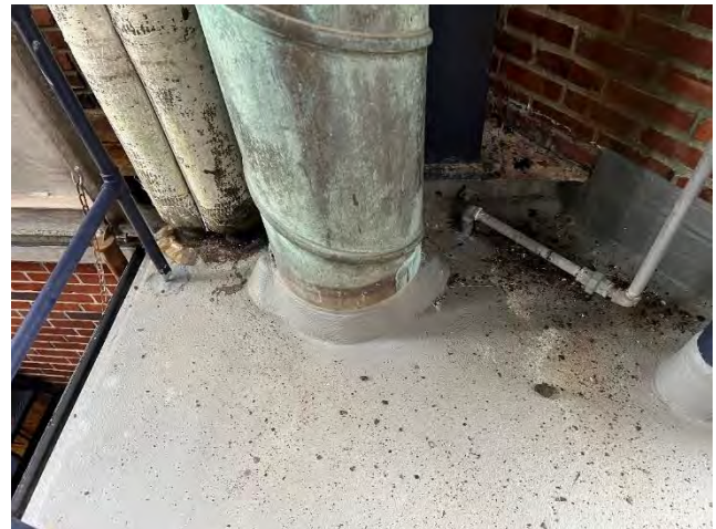
Figure 14 Examples of roof penetrations
