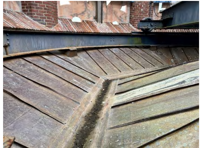
5 Upper roof slopes to an internal gutter
