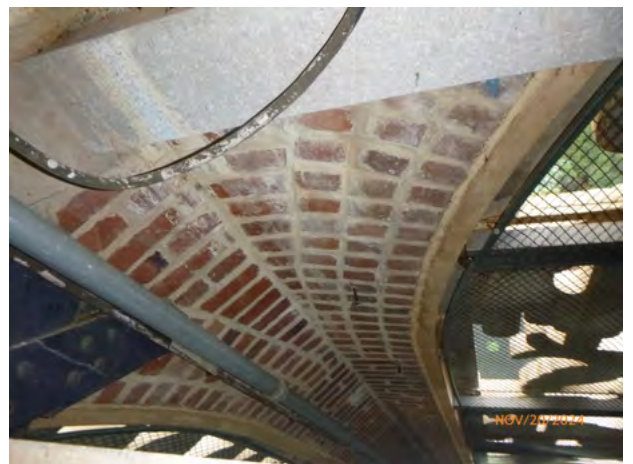
542-171 Brick_SoilStain Paint 2024-2.jpg
