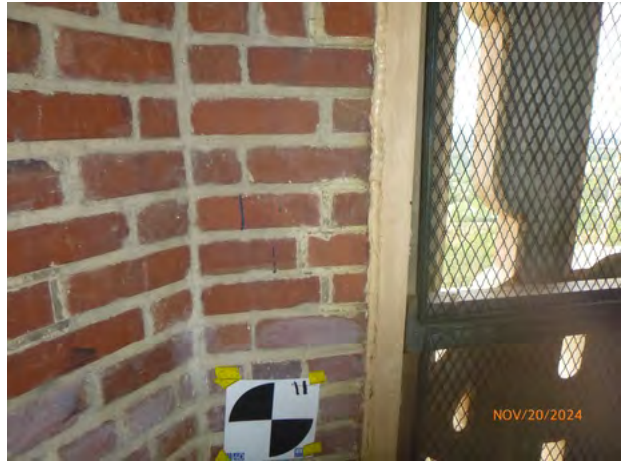
757-150 Brick_Repair Patch Sound 2024-1.jpg
