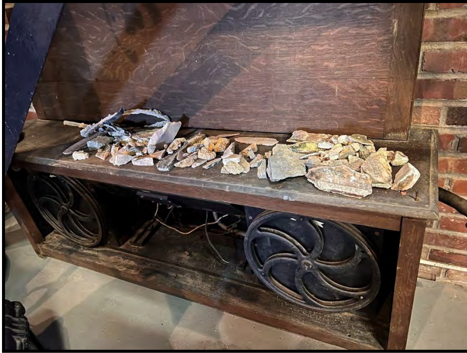
Figure 33 Loose material removed from the tower façade by Vertical Access
