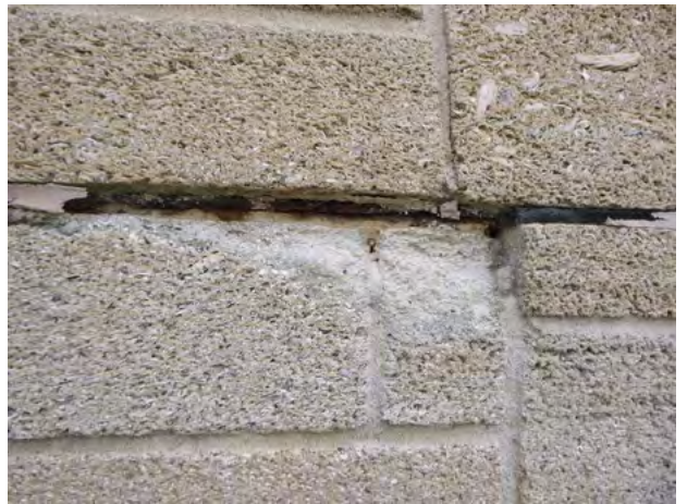
149-91 Stone_Spall Removed + Steel 2024-2.jpg
