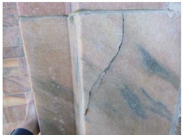
35-114 Stone_Spall Bonded 2024-1.jpg
