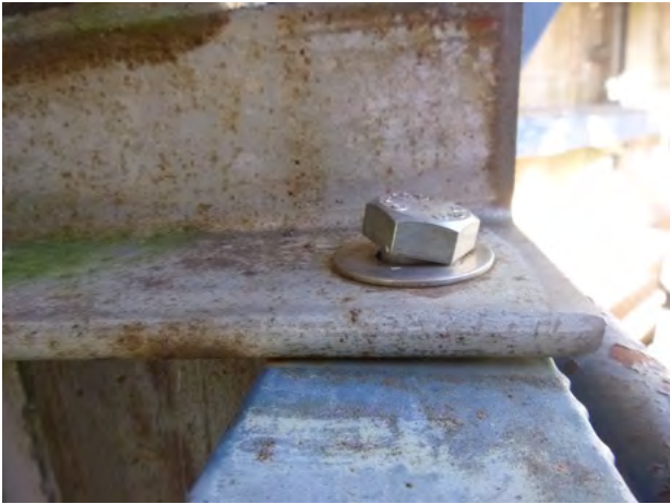
649-189 ArchMetal_Note Photo-connections askew 2024-2.jpg
