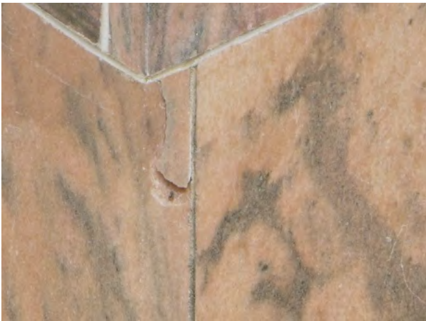
282-134 Stone_Spall Bonded 2024-1.jpg
