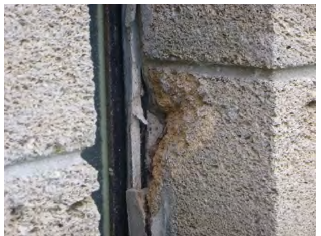
51-87 Stone_Spall Removed + Steel 2024-4.jpg
