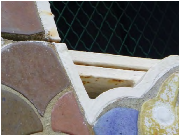
186-168 ArchMetal_Corrosion Surface 2024-1.jpg
