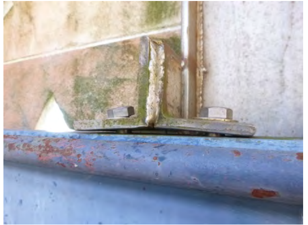
649-189 ArchMetal_Note Photo-connections askew 2024-3.jpg
