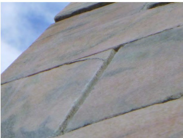
42-152 Stone_Spall Bonded 2024-1.jpg
