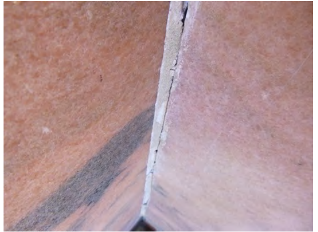
639-194 Stone_Joints Mortar Failed 2024-2.jpg
