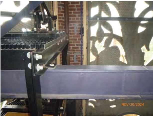
658-146 Brick_Unsecured Missing 2024-1.jpg
