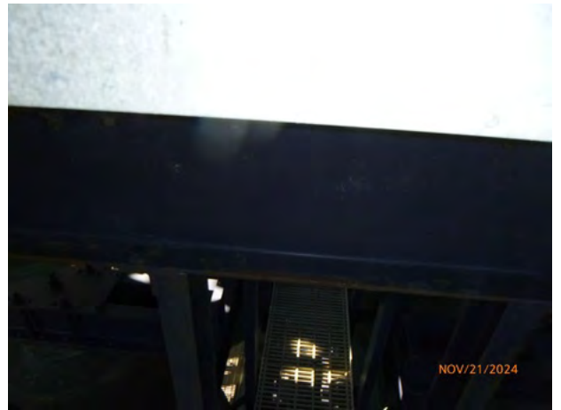
562-170 ArchMetal_Coating Coating Failed 2024-4.jpg
