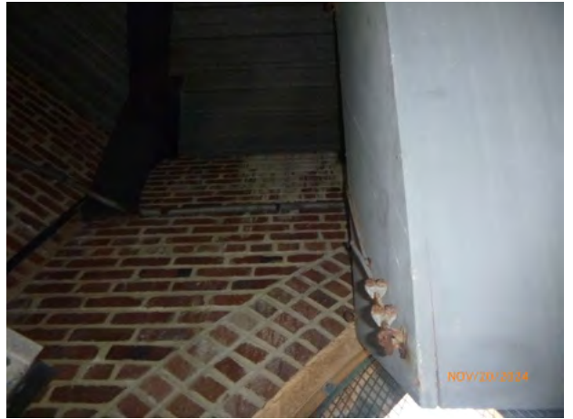
558-178 Brick_SoilStain Paint 2024-1.jpg
