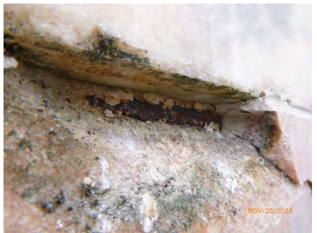
132-71 Stone_Spall Removed + Steel 2024-3.jpg
