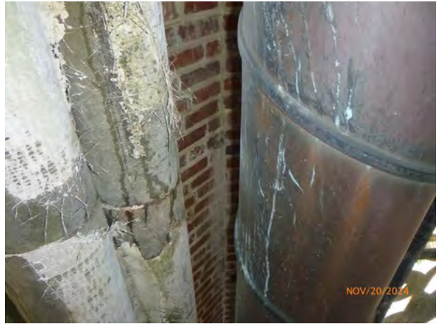
756-166 Brick_SoilStain Paint 2024-1.jpg
