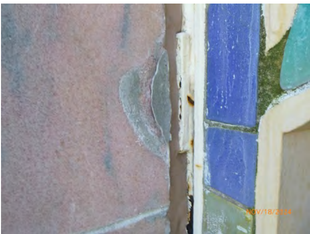
36-154 Stone_Spall Bonded 2024-1.jpg
