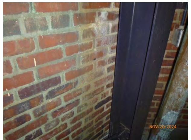
656-140 Brick_SoilStain Paint 2024-2.jpg
