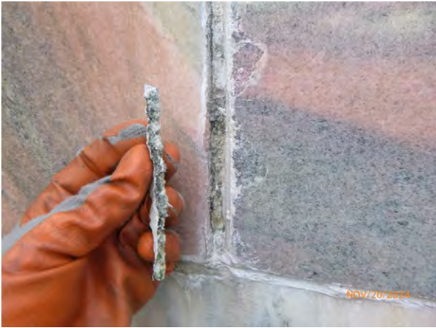
132-181 Stone_Joints Mortar Removed 2024-3.jpg
