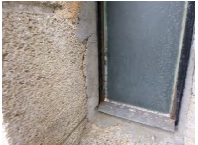
50-87 Stone_Spall Bonded 2024-3.jpg
