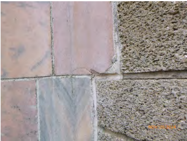
133-46 Stone_Spall Bonded 2024-2.jpg
