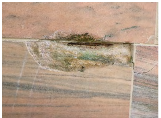
160-46 Stone_Spall Removed + Steel 2024-2.jpg
