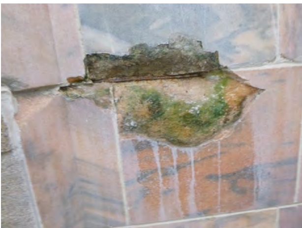
141-69 Stone_Spall Removed + Steel 2024-2.jpg
