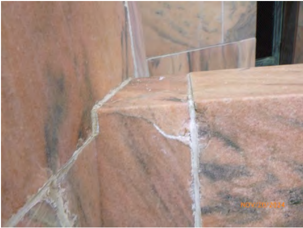
133-141 Stone_Spall Bonded 2024-1.jpg
