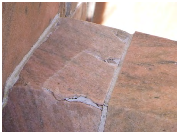
334-142 Stone_Spall Bonded 2024-1.jpg
