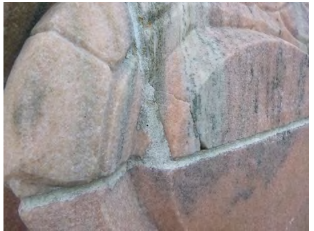
142-194 Stone_Spall Bonded 2024-1.jpg
