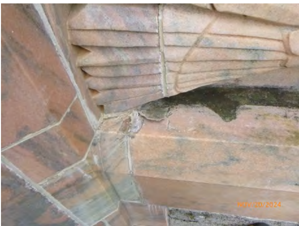
60-139 Stone_Repair Patch Removed 2024-1.jpg
