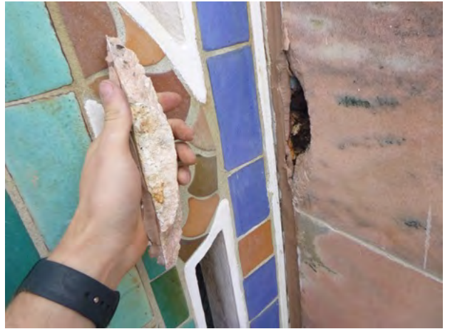
194-154 Stone_Spall Removed + Steel 2024-3.jpg
