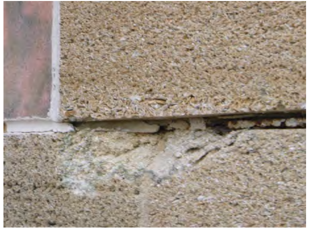
146-91 Stone_Spall Removed + Steel 2024-1.jpg
