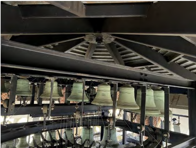
4 Underside of upper roof
