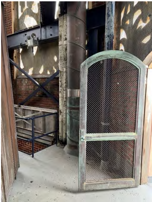
9 Lower roof connection to balcony
