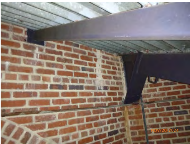
657-178 Brick_SoilStain Paint 2024-1.jpg
