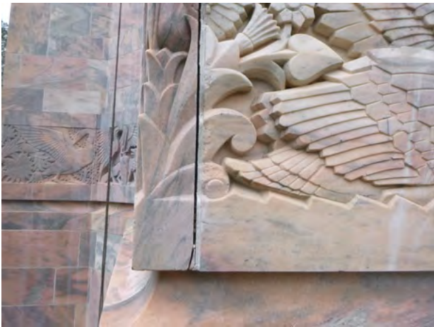
134-30 Stone_Displacement Horizontal 2024-3.jpg
