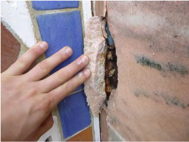
194-154 Stone_Spall Removed + Steel 2024-2.jpg
