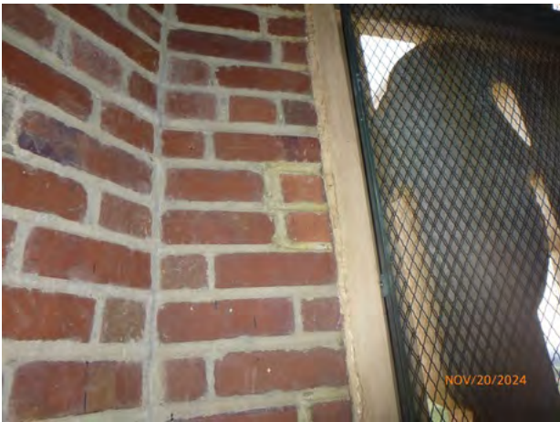
757-152 Brick_Repair Patch Sound 2024-1.jpg
