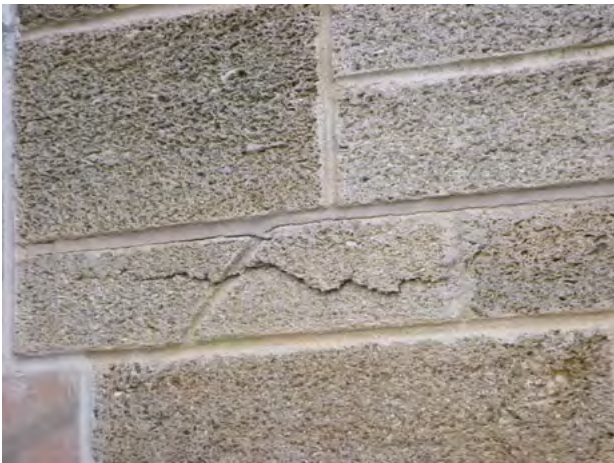
46-101 Stone_Spall Bonded 2024-1.jpg
