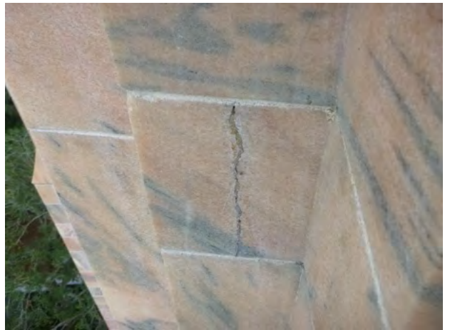
134-129 Stone_Crack Repair sound 2024-1.jpg
