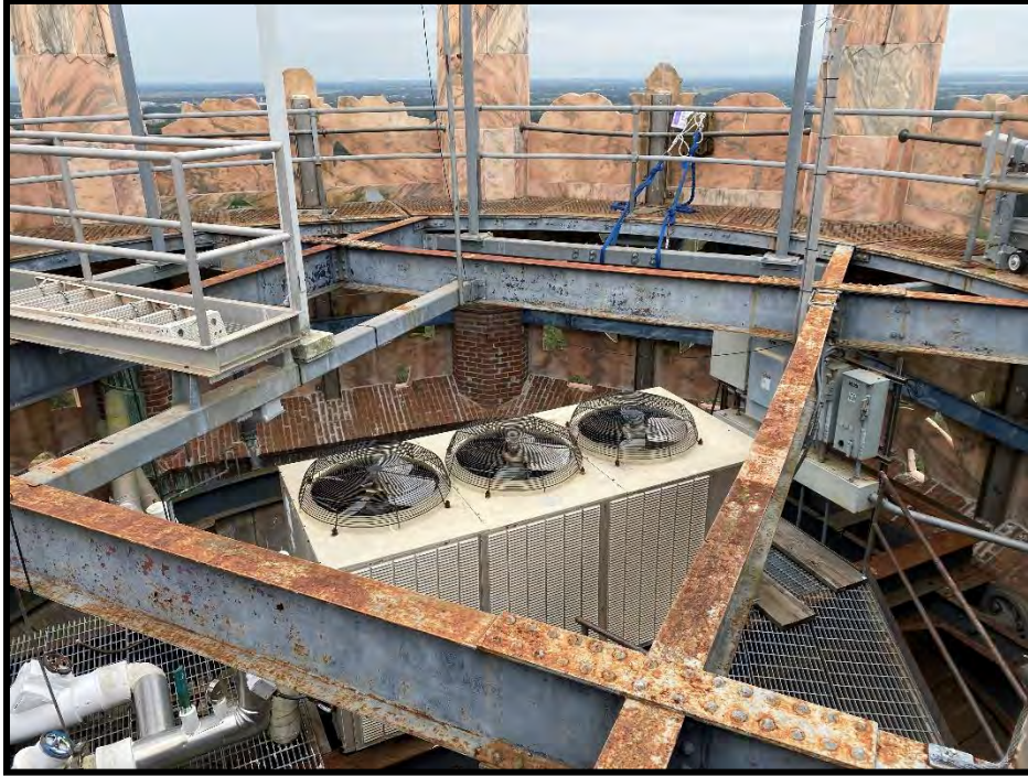
Figure 17 Exposed steel framing above the roof level
