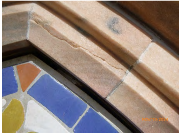
239-178 Stone_Spall Bonded 2024-4.jpg
