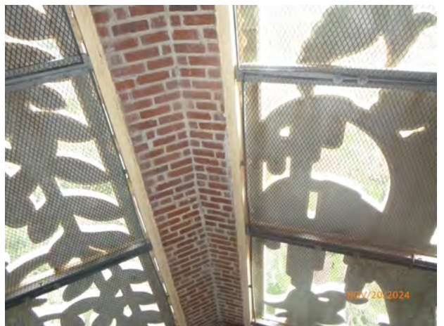
745-167 Brick_SoilStain Paint 2024-1.jpg
