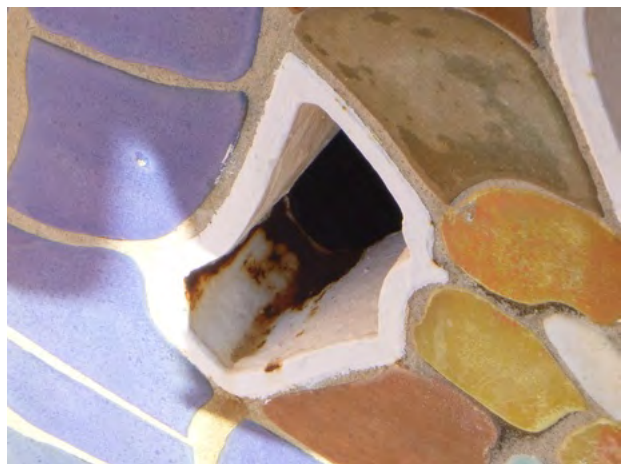
285-145 ArchMetal_Corrosion Surface 2024-1.jpg
