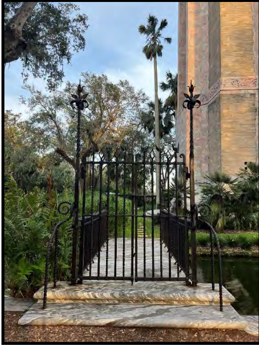
Figure 9 Gate and bridge over the tower moat
