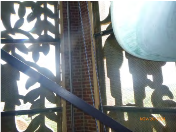
542-157 Brick_SoilStain Leached Salts 2024-1.jpg
