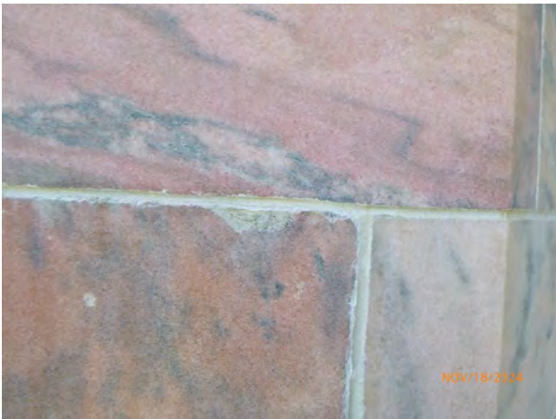
34-172 Stone_Repair Patch Sound 2024-1.jpg
