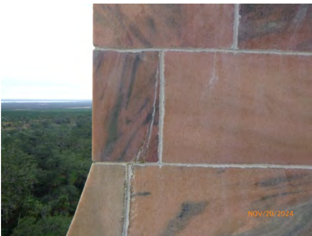
130-123 Stone_Crack Repair sound 2024-1.jpg
